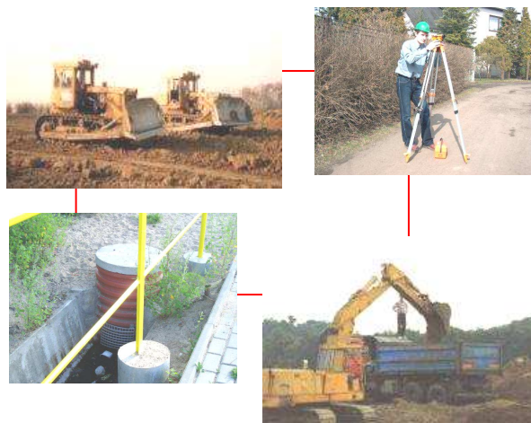
Photo. Road and hydro-engineering
