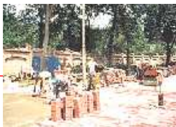
Photo. Paving works
